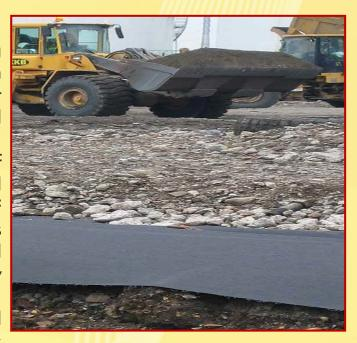
foundations, embankments and coastal defences. Woven geotextiles provide a cost effective solution for the separation of granular fill materials and for the provision of sub structure support. The most common application is for the use as a separating layer beneath roads, helping to prevent rutting through separation and tensile support.
