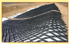
infilled, provides a semi-rigid foundation. Traffic loads are distributed laterally, reducing rutting and assisting in the retention of infill materials.
