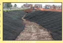
layer, helping to retain good soil and seed on steep slopes. Constructed from multiple layers of high tensile polyethylene, it traps soil particles in position helping to encourage seed germination.
